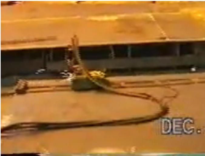
Some plates were three inches thick. Too thick for shears. These thicker plates were removed from the line at some point and taken to the torch cutting areas. The picture at the left shows a cutting torch on its little track cutting a plate. Raul Maestro was one of the Puerto Rican torch operators. We will meet him later in one of my stories of Sunday labor.
